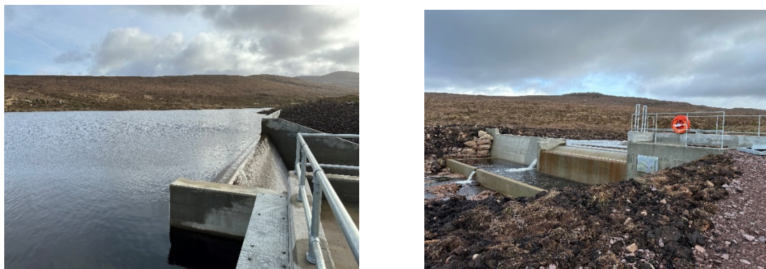
Figure 2 – intake to penstock from Reservoir
