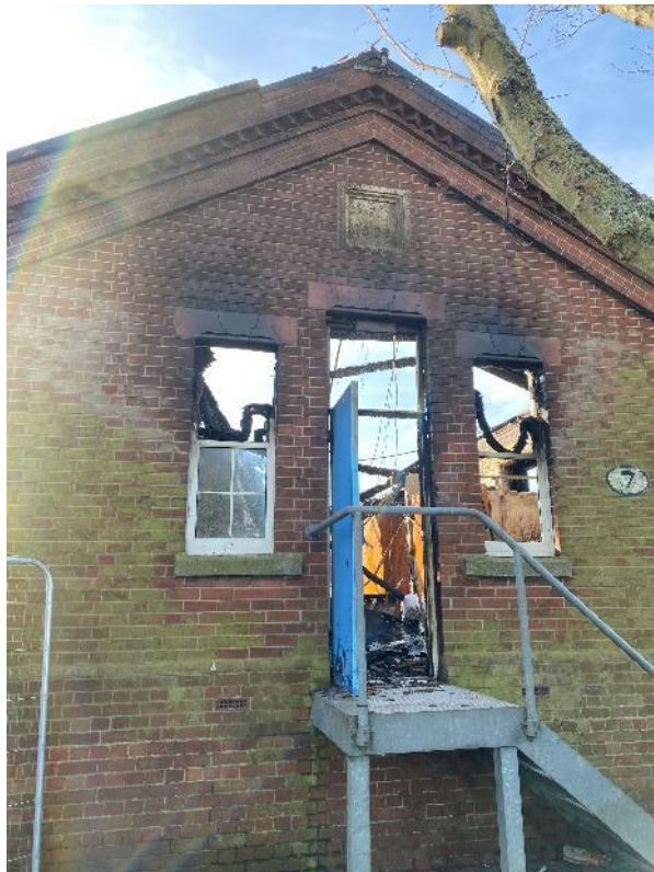
4. Stand back view of rear elevation
