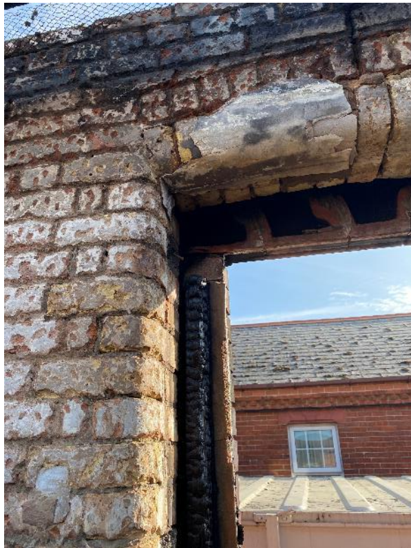
8. Typical window reveal and cavity
