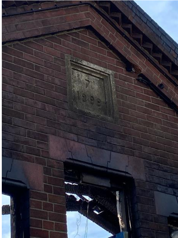
3. Gable to rear (north elevation) of building
