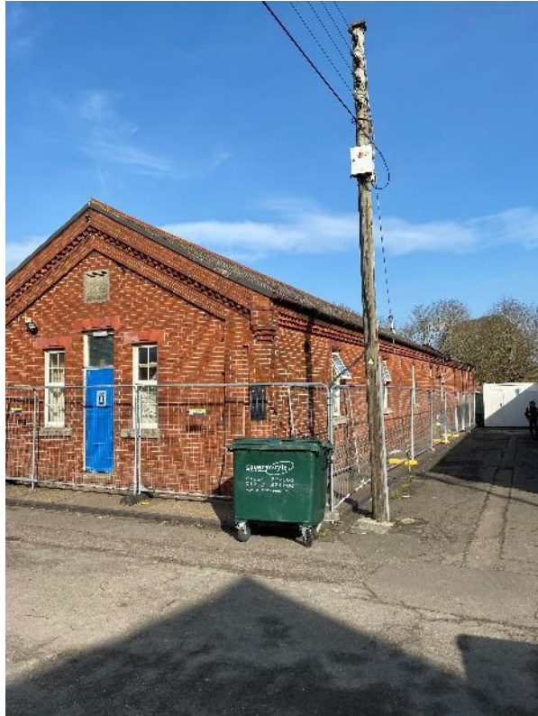
1. Front (south elevation) of building
