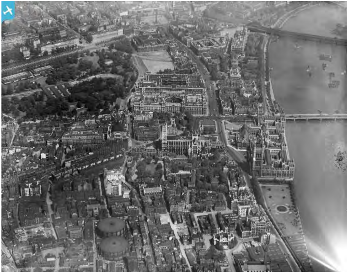
Figure 4.2 Historic Context – Aerial Photographs
