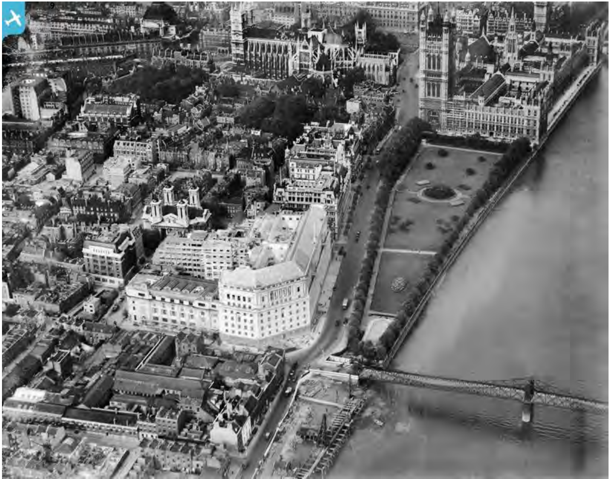
Figure 4.2.1 Historic Context – Aerial Photographs
