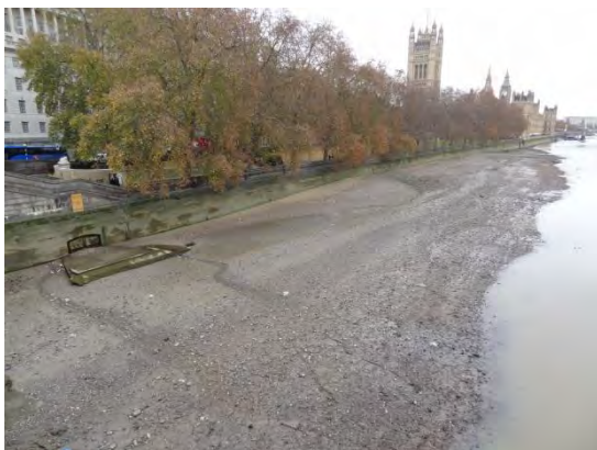
View from Lambeth Bridge including foreshore (outlet under bridge steps visible)
