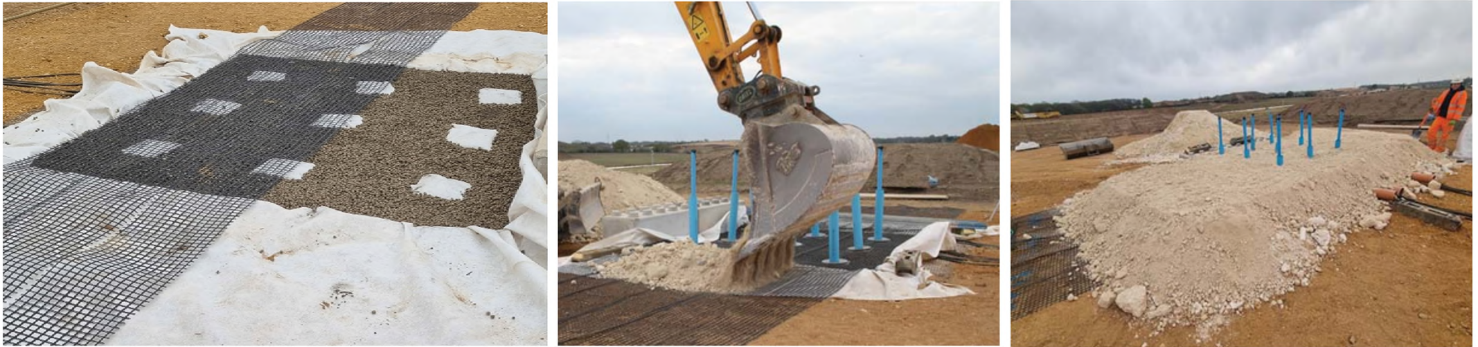
(c) Construction of site trial – Sensorgrid over water bags with backfill above
