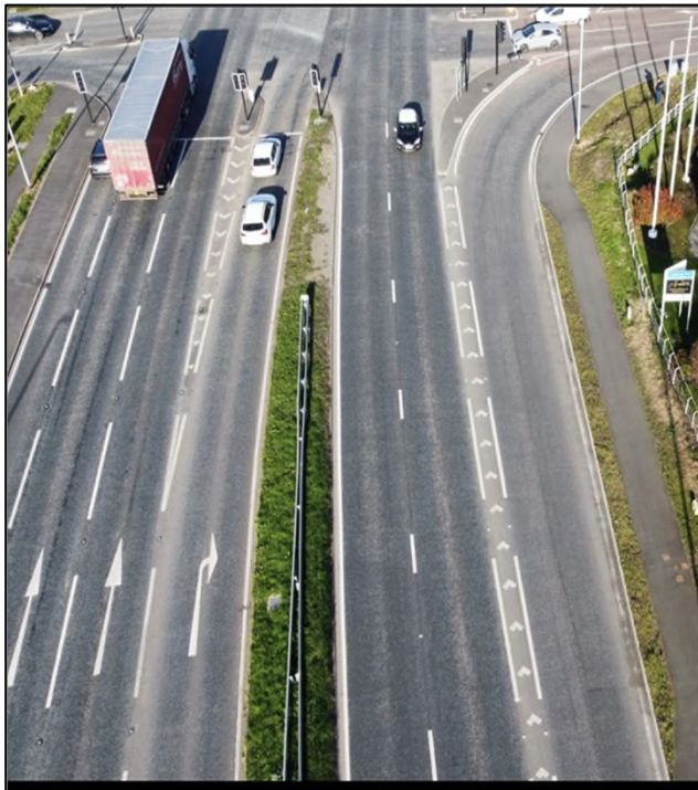
Fig 1 - The new eastbound & west bound slip roads
