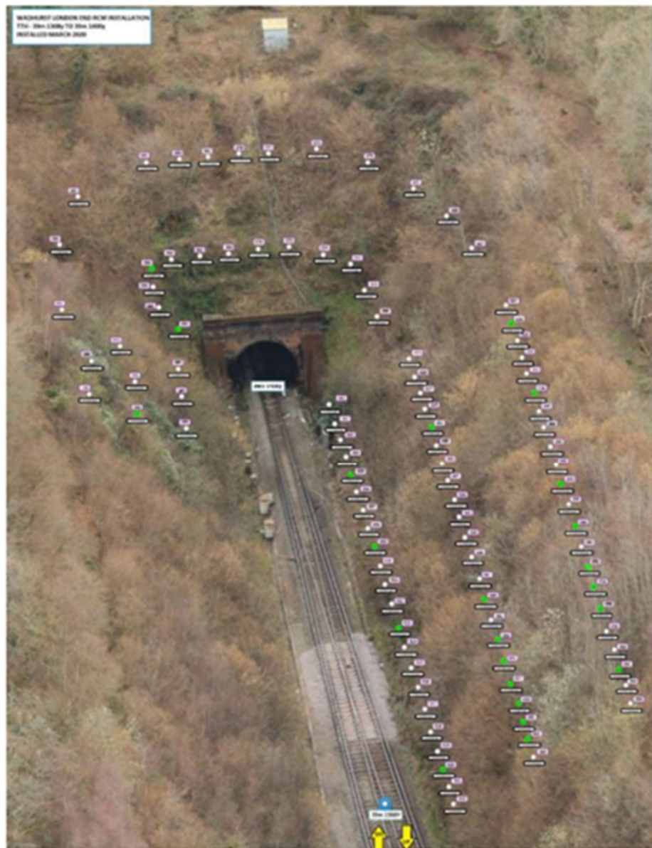
Figure 10.3: Wireless tiltmeters around a tunnel portal (Network Rail presentation, 9 October 2020)
