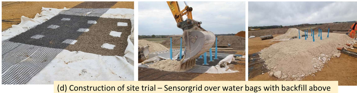
Fig.1 Field simulation of ground movement: (a) Schematic diagram of field experiments at the initial stage; (b) Schematic diagram of field experiments when bags deflated; (c) results for deflation of cell A2, small displacements results, (d) Construction of field experimental setup (after Xu et al, 2022)
