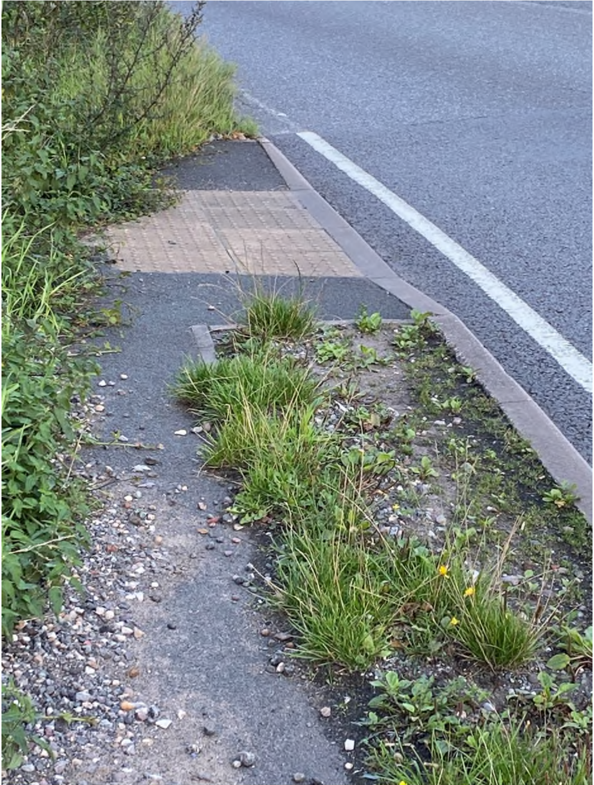
Current pedestrian crossing picture 2
