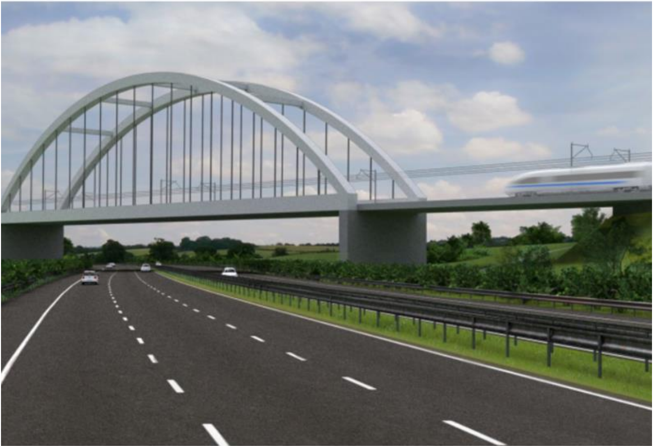
Figure 5: Visual representation of the HS2 Phase 2a M6 Meaford viaduct incorporating a single span bridge over the M6 motorway
