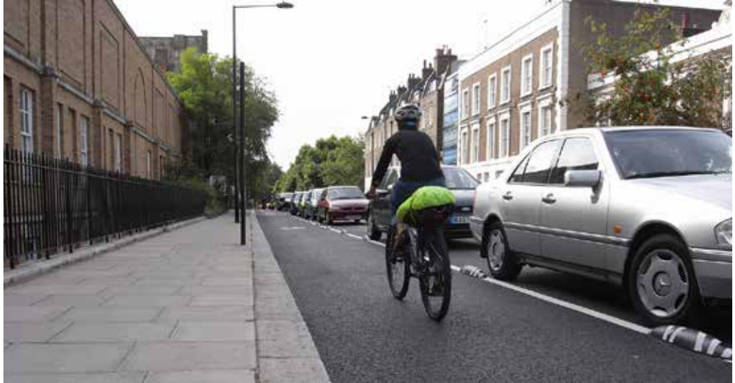
Photo 6.9 – Light segregated cycle track with wand at start, Salford, Greater Manchester (Note – only one lane marking, outside the raised features, should be used).
